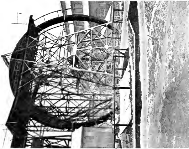
WHEEL FOR LIFTING CRUSHED ROCK, WHICH HAS RUN OVER THE BATTERY PLATS, TO THE CYANIDE TANKS, KLEINFONTEIN MINE.
